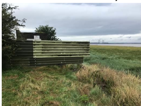
Barrier that westernmost sentry box
